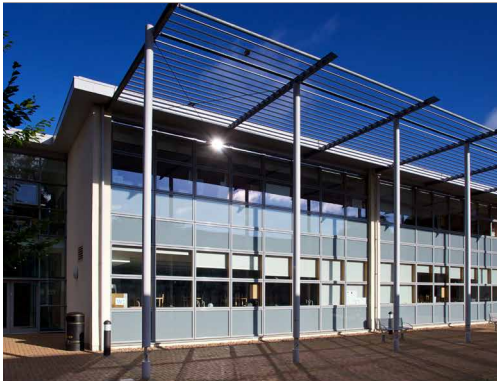
LES Chemistry Building Loughborough
