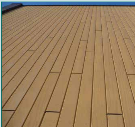
ACCOYA AS CLADDING PHOTO: © TITAN WOOD LTD
