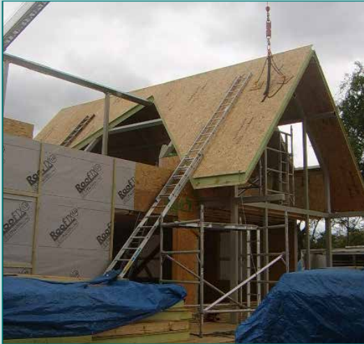
SIPS PANELS BEING ERRECTED IN A DOMESTIC SITUATION PHOTOS COURTESY SIPS UK LTD.
