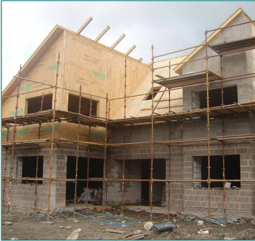
SIPS PANELS BEING ERECTED IN A DOMESTIC SITUATION PHOTOS COURTESY SIPS UK LTD.
