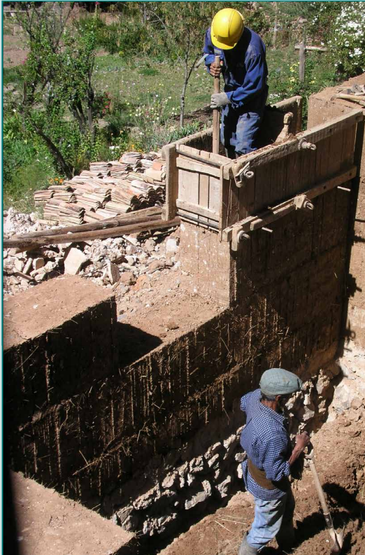
RAMMED EARTH WALLS AND FLOORS UNDER CONSTRUCTION IN PERU: JYB DEVOT, CC BY-SA 4.0, VIA WIKIMEDIA COMMONS
