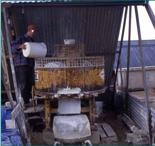
LIME MORTAR BEING MIXED PHOTO: JJ SHARPE
