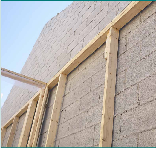
CONCRETE BLOCKWORK UNDER CONSTRUCTION PHOTOS.COM WEBSITE
