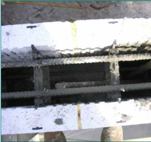
A CLOSE-UP TOP VIEW OF ICF BLOCKS UNDER CONSTRUCTION PHOTO: MIKEOG39 - HTTP://WWW.WISEHOMEDESIGN.COM
