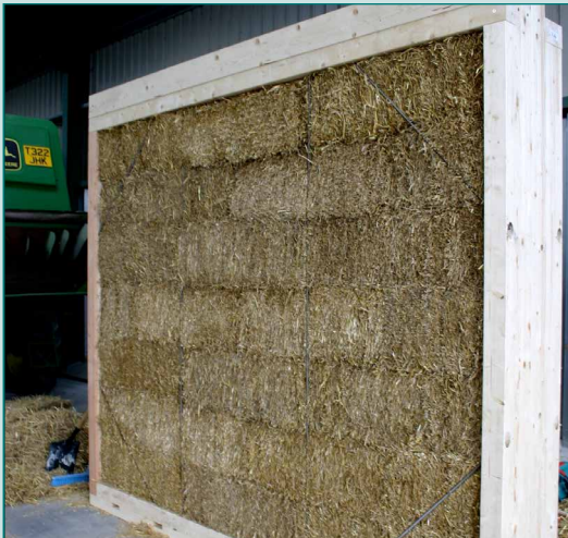
MODCELL PANELS UNDER CONSTRUCTION PHOTO: MODCELL (WWW.MODCELL.CO.UK)
