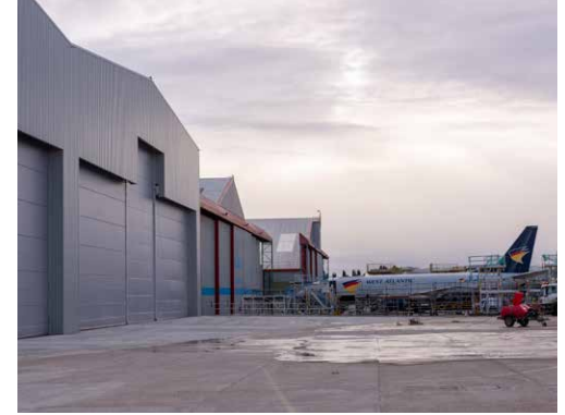
Airport Hangar Norwich
