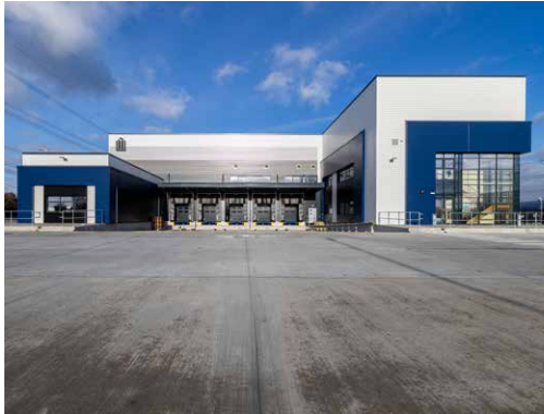
DPD Barge Way Sittingbourne
