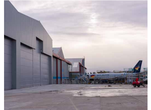
Airport Hangar Norwich
