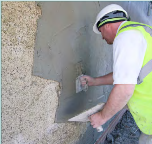
LIME RENDER BEING APPLIED OVER HEMCRETE BASE PHOTO: COPYRIGHT © 2000-2009 LIME TECHNOLOGY LIMITED
